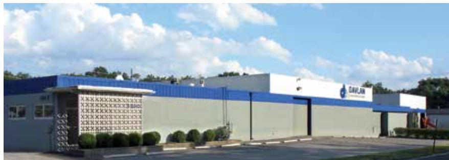
Above: Davlan Engineering's building. The firm has added on six times.
